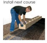
Step 3: Stack the next course of block on top of the grid, so that the blocks are offset from the blocks below. Pull on the back of the grid to remove any slack and stake in place.
